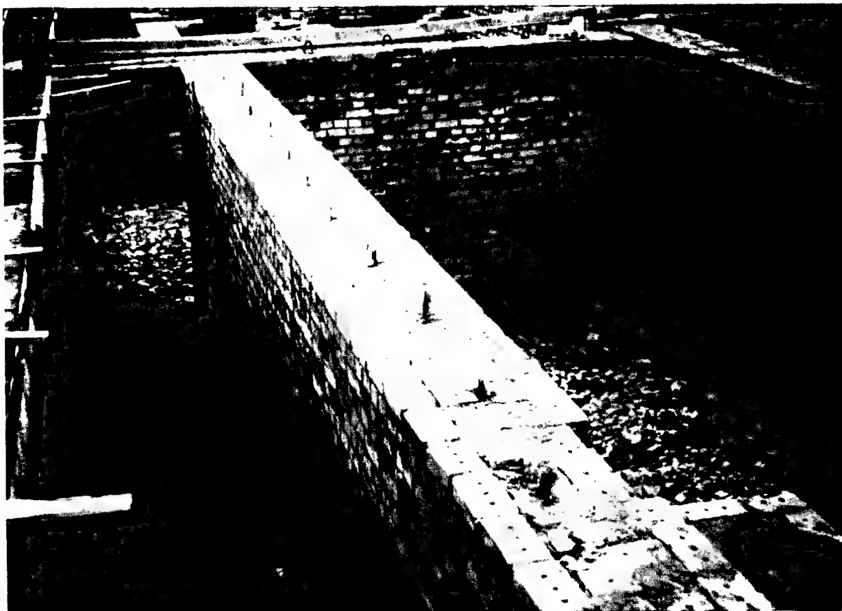
Figure 12 COMPARTMENTIZED BASEMENT AIR-RAID SHELTER Kiev, USSR
